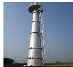
M S CHIMNEY
